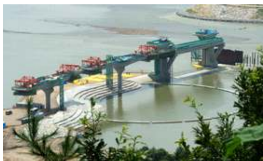
Fig. II-1-5 Epo small dam in Han river
