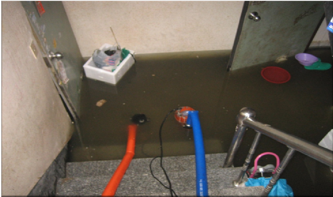
Fig. II-1-8. Basement of a house flooded due to the heavy rains on 21 September 2010 in Seoul, South Korea.
