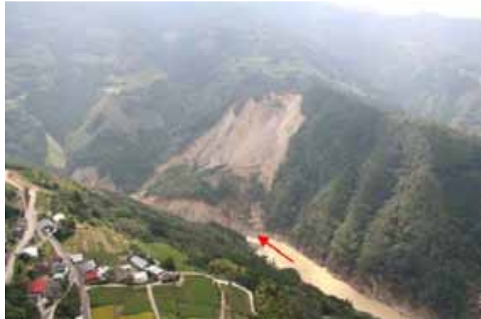
Figure 13. Example of a natural dam – a sediment-related disaster caused by a deep rapid landslide (Mimikawa River, Miyazaki Pref.)
