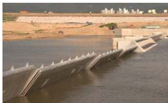
Fig. II-1-6 Gunnam small dam in Gum river
