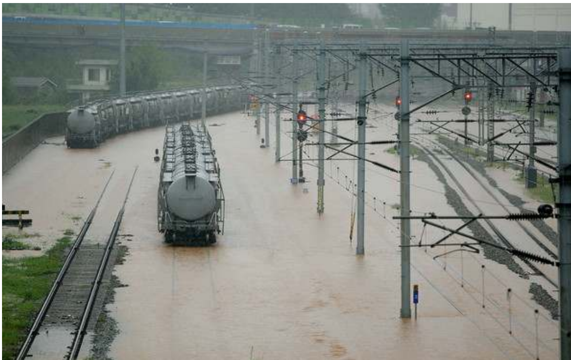
Fig. II-1-15. A subway station flooded due to the heavy rains on 21 September 2010 in Seoul, South Korea.
