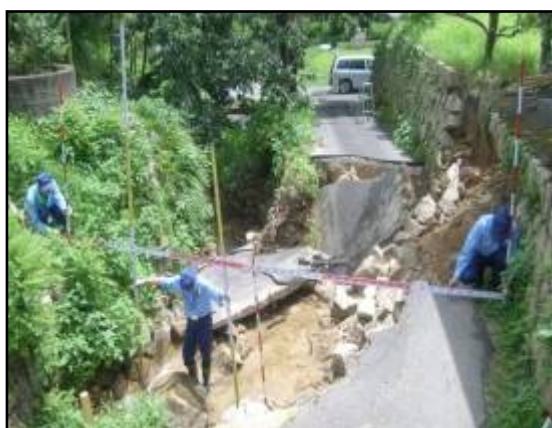
Figure 10. Damage assessment on the ground
